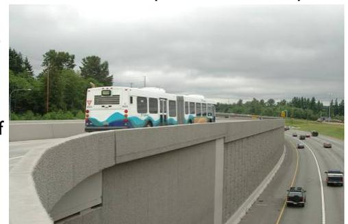
*Ash Way Direct Access Ramps to I-5 were designed to only allow transit vehicles due to close proximity to other interchanges and the desire to limit merging and weaving.*
